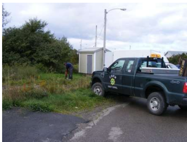
Figure 2. Abandoning old well October 2008, new treatment building in background.
