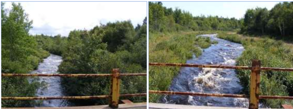
Figure 3. Spillway channel September 2008 on left and September 2012 on right
