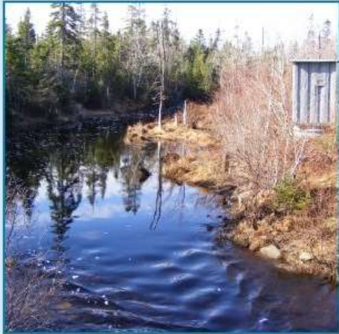
This hydrometric station measures MacAskill's Brook water flow into the reservoir.
