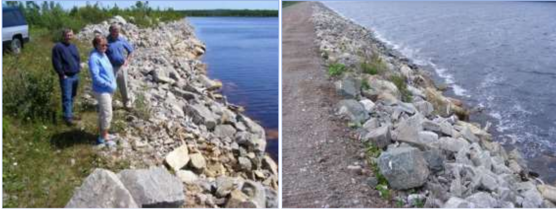
Figure 8. Before and after rip rap repairs July 2009 and July 2011
