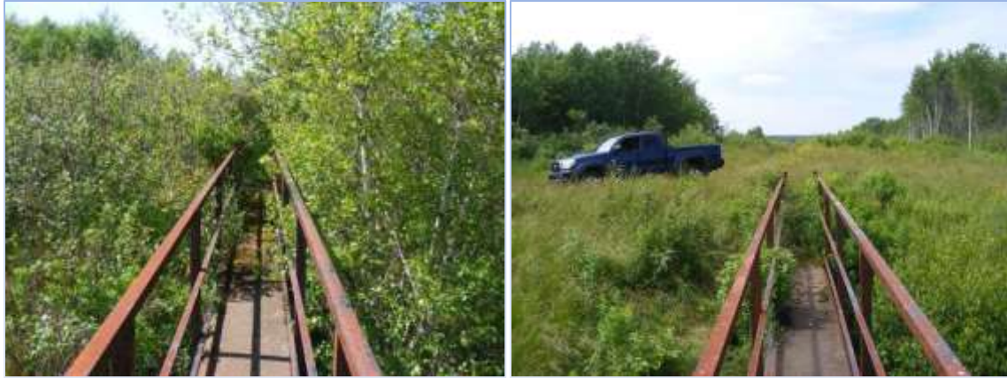
Figure 6. Top of dam from spillway June 2009 on left and July 2013 on right
