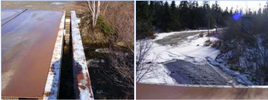
Figure 13. Bridge over MacAskill Brook on old Cow Bay Road
