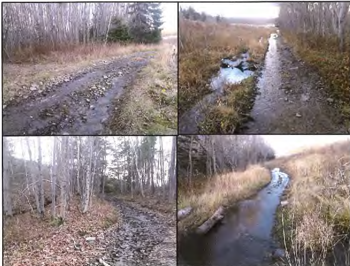
Photo 17-20. Four photos show unrestricted flows in the right of way zone of Highway 125. Flows were observed on the afternoon of November 26, 2019, 24h after the rainfall (17mm) of the previous day. These are normal flows for this time of year given historical rainfall data for Sydney These flows would have been an order of magnitude greater on the flood event of October 2016. Figures 12-14 show opportunities to restrain and infiltrate this runoff before it reaches the brooks.
