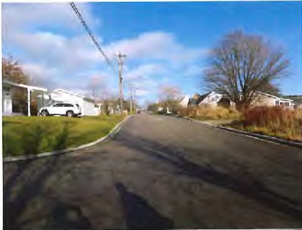
Photos 9 and 10: Herbert Street. The long (800m) urban slope of Herbert Street and further up to Lisgard St, flows down pavement (Photo 9) and over the embankment (Photo 10) into the back of the Centennial Arena (Photo 11).
