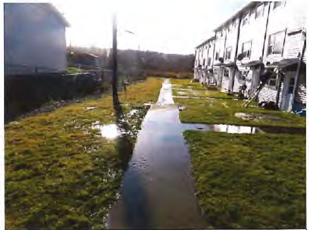
Photo 13 and 14. Urban rubble in front of housing complex (13). Overloaded storm sewer flows down walkway of Dahlia Terrace (14) the day after a rain. Wetland restoration and drainage redirection can alleviate this chronic neighbourhood issue.
