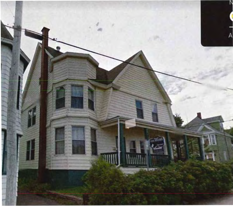
Photograph taken in 2012 showing the east and north faces of 26 Archibald Avenue, North Sydney, B2A 2W3.
