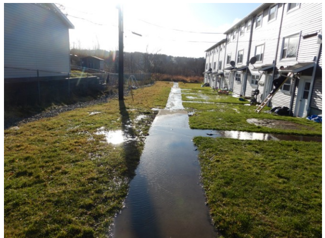
Photo 13 and 14. Urban rubble in front of housing complex (13). Overloaded storm sewer flows down walkway of Dahlia Terrace (14) the day after a rain. Wetland restoration and drainage redirection can alleviate this chronic and unhealthy neighbourhood issue.
