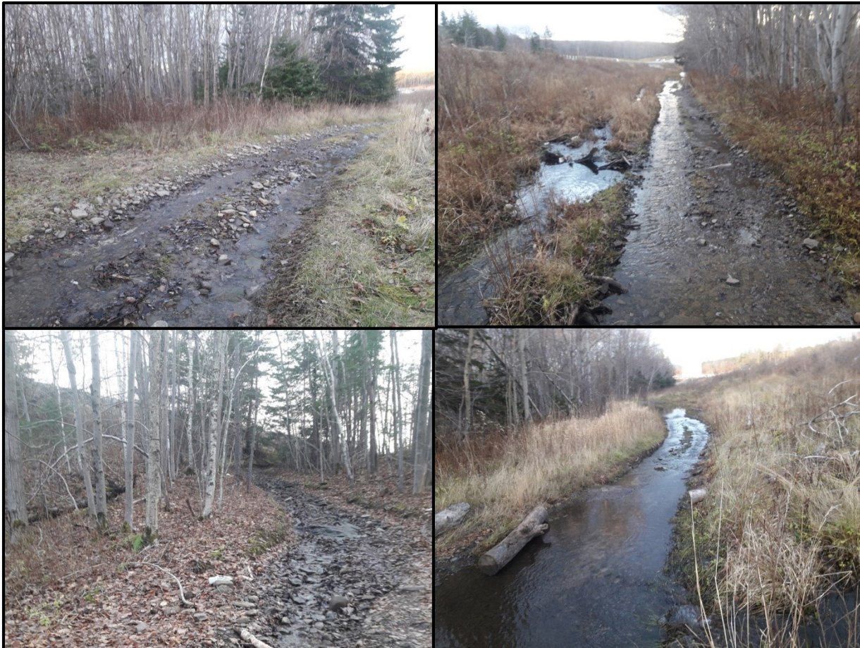
Photo 17-20. Four photos show unrestricted flows in the right of way zone of Highway 125. Flows were observed on the afternoon of November 26, 2019, 24h after the rainfall (17mm) of the previous day. These are normal flows for this time of year given historical rainfall data for Sydney. These flows would have been an order of magnitude greater on the flood event of October 2016. Figures 12-14 show opportunities to restrain and infiltrate this runoff before it reaches the brooks.
