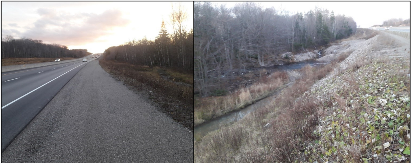
Photo 15 and 16. Peacekeepers Highway 125. At left (12), shows the highway divider, the paved twin lane highway, the gravel verge and the embankment above the surrounding woodland. At right (16) is the highway edge and the downstream flow from Gilholmes Lake stream. Note the central stream and water in the ditch zone that contributes to that stream flow. Figures 8-10 give example cases of how such flows can be intercepted and infiltrated relatively cheaply using berms and diversions at the woodland edge.
