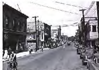
1965, the heritage India Building built in 1929 photo credit: Beaton Institute
