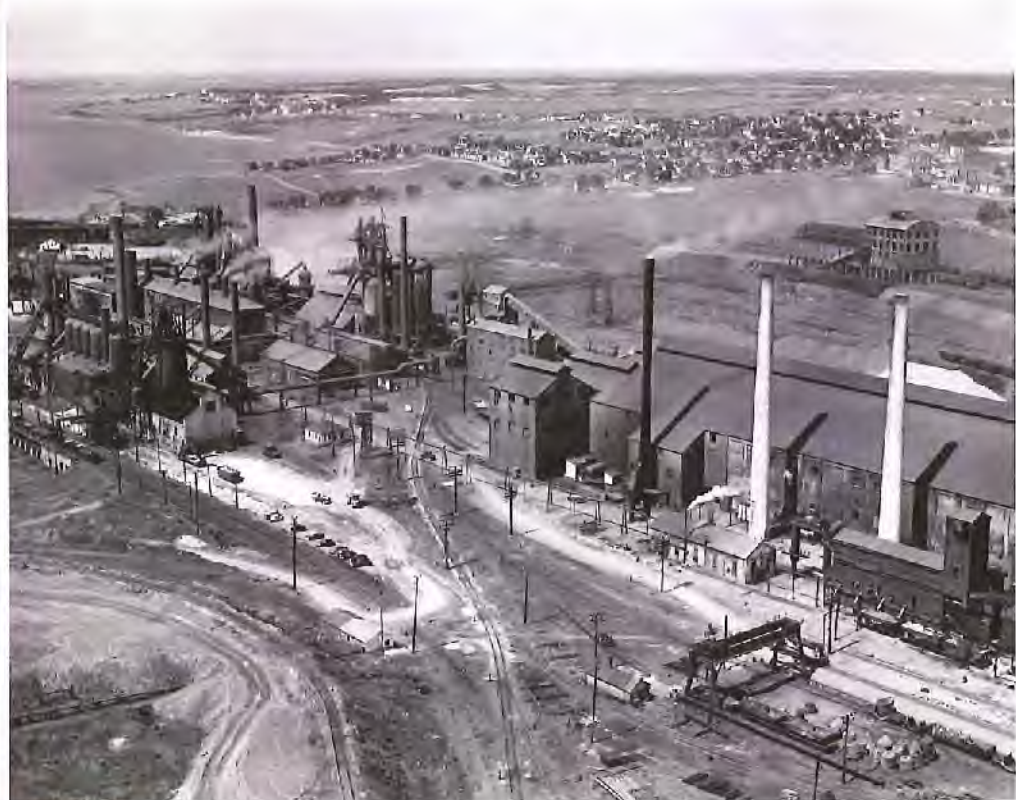
Industrial steel plant in Sydney photo credit: Nova Scotia Archives NSIS no. 14419
