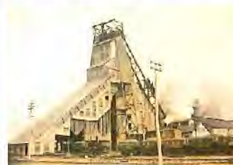
ca. 1960, Glass Bay No. 2 colliery photo credit: Boston Institute 77-691-851
