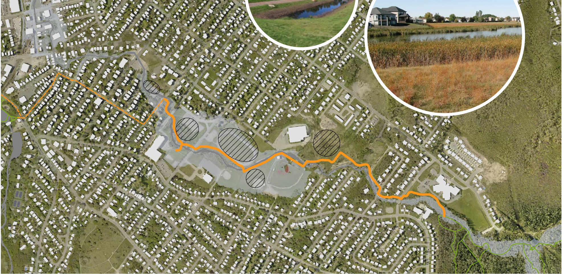
Naturalized wetland stormwater retention basin (Winnipeg, MB)
