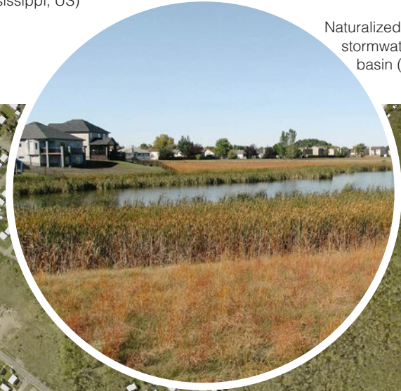
Typical stormwater retention basin (Mississippi, US)
