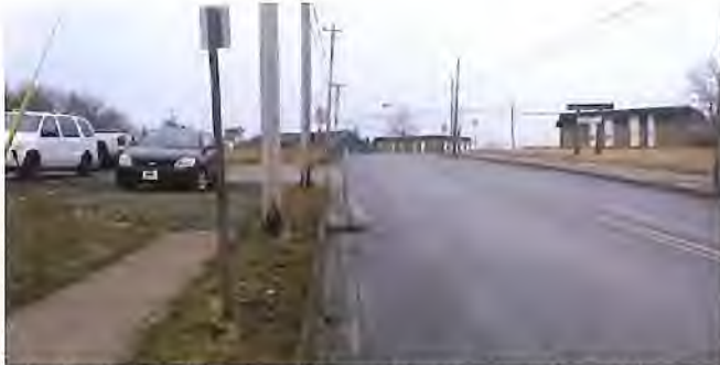
Photo 2: Looking south on King Street from Access Location B. The site's existing driveway is visible on the left.
