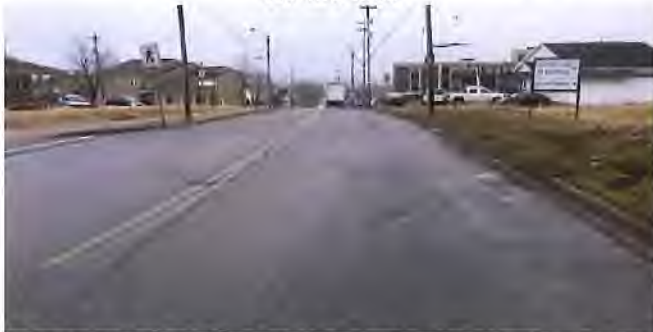
Photo 4: Looking north on King Street toward Access Location B.
