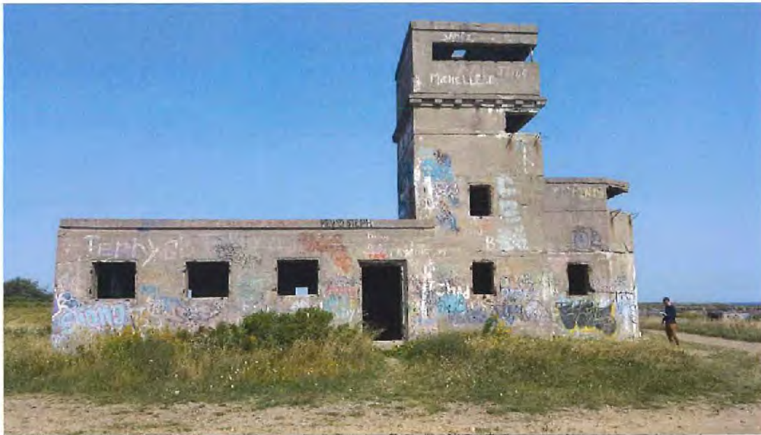
Exterior side elevation view of Battery Command Post
