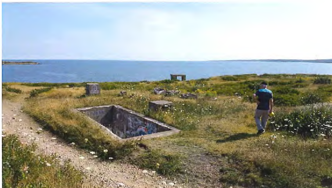
Open stairwell to underground Power House
