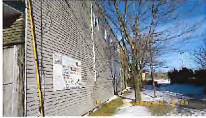
Side of Building adjacent to CIBC
