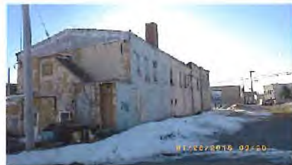
Back of Building Depicts General Disrepair of Building
