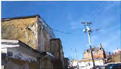
NSP Wires connected to building
